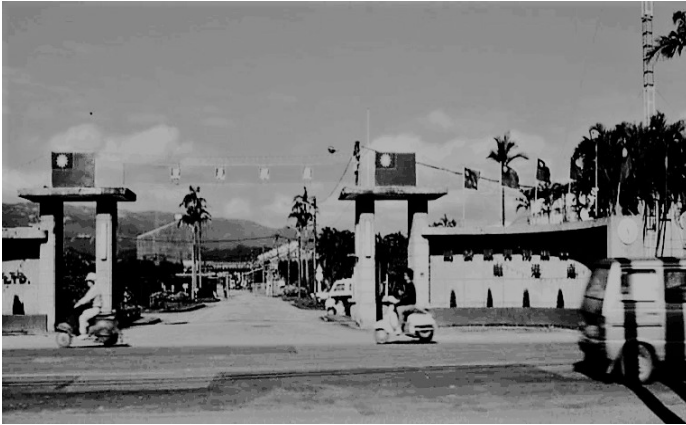
Figure 1. The main gate of Nangang Factory, the Taiwan Fertilizer Company.
